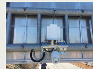
돌발상향검지시스템(AIDS) Automatic Incident Detection Systems
