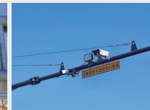
차량검지기(VDS) Vehicle Detection System
