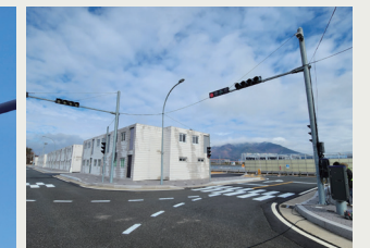
교통신호제어기(TSC) Traffic Signal Controller
