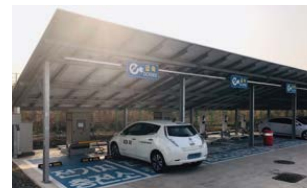
DC CHAdeMO type bi-directional electric vehicle charger(2 units) (Charge : 50kW / Discharge : 20kW)
